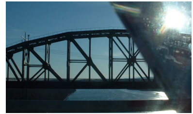
Figure 6.4: Many bridges, especially old train bridges, are essentially trusses. Here’s one that is partially obscured by the truss on a nearby car bridge.
