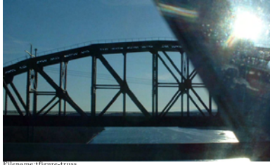
Figure 5.4: Many bridges, especially old train bridges, are essentially trusses. Here's one that is partially obscured by the truss on a nearby car bridge.
