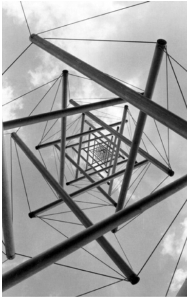
Figure 5.11: Sometimes trusses are used only because they look nice. The tensegrity structure ‘Needle Tower’ was designed by artist Kenneth Snelson and is on display in the Hirshhorn Museum in Washington, DC. It doesn’t hold up anything but itself. Here you are looking straight up the middle. (courtesy Christopher Rywalt)
