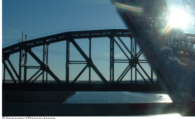
Figure 5.4: Many bridges, especially old train bridges, are essentially trusses. Here's one that is partially obscured by the truss on a nearby car bridge.
