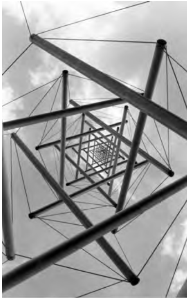
Figure 6.11: Sometimes trusses are used only because they look nice. The tensegrity structure ‘Needle Tower’ was designed by artist Kenneth Snelson and is on display in the Hirshhorn Museum in Washington, DC. It doesn’t hold up anything but itself. Here you are looking straight up the middle. (courtesy Christopher Rywalt)
