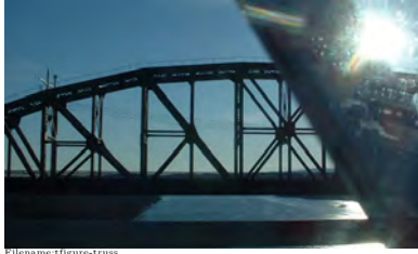
Figure 6.4: Many bridges, especially old train bridges, are essentially trusses. Here's one that is partially obscured by the truss on a nearby car bridge.
